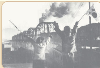
Recovering Han River Bridge in Seoul
