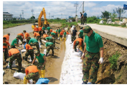
Repairing waterways in fields
